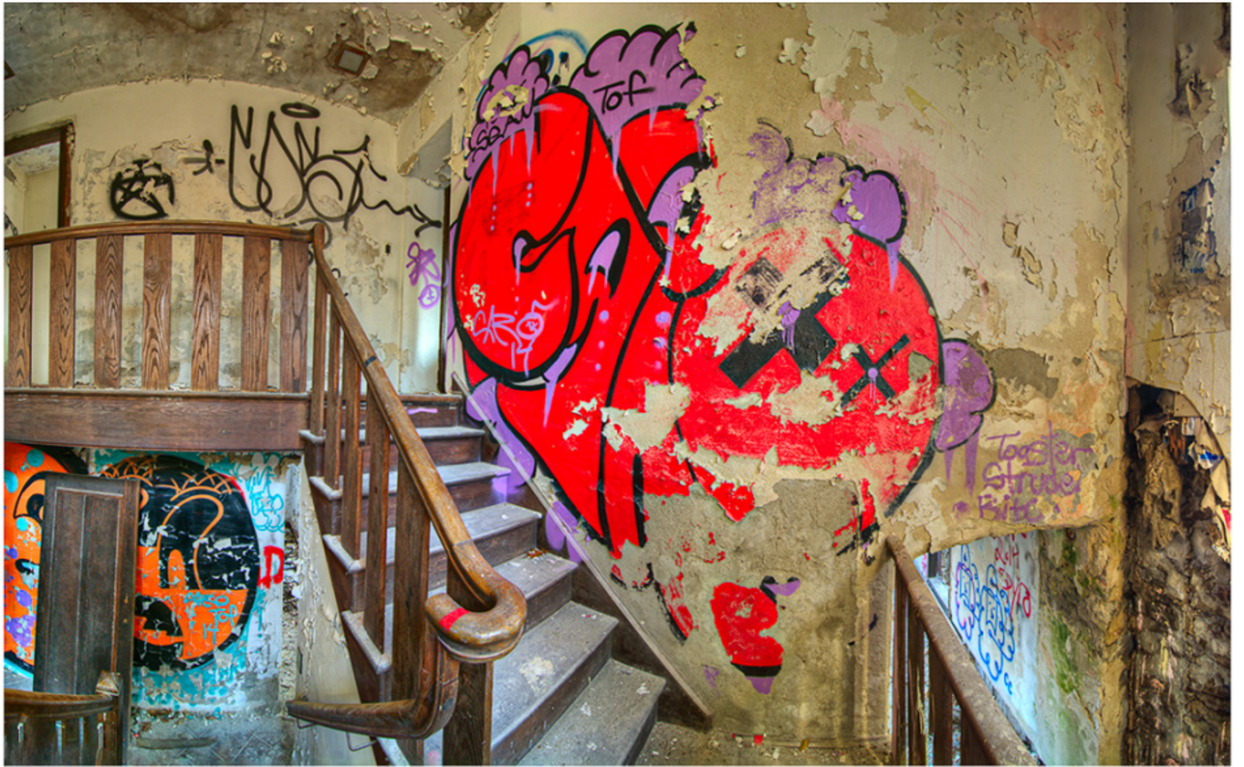
Staircase to the second floor.
